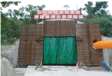
图 6 洞口飞石防护装置 Fig. 6 Protective device for flying rocks at the entrance
