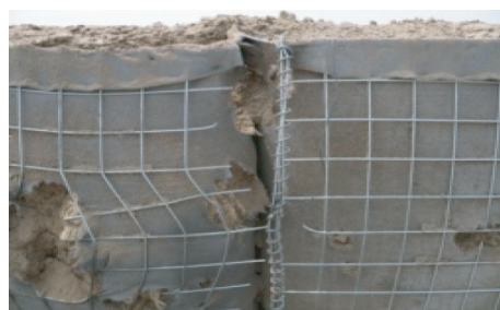
(c) 钢质网片变形、脱焊
